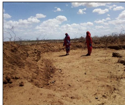
Process of digging pans for water storage
